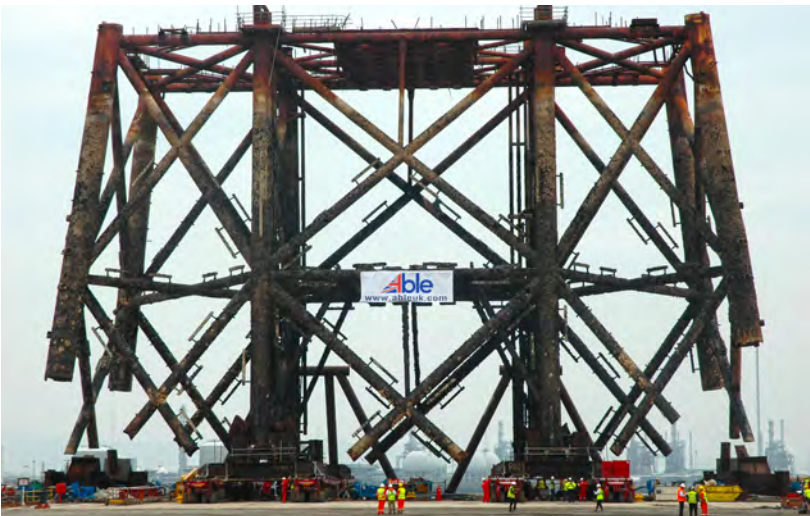
BP North West Hutton Jacket SPMT Movement at ABLE Seaton Port
